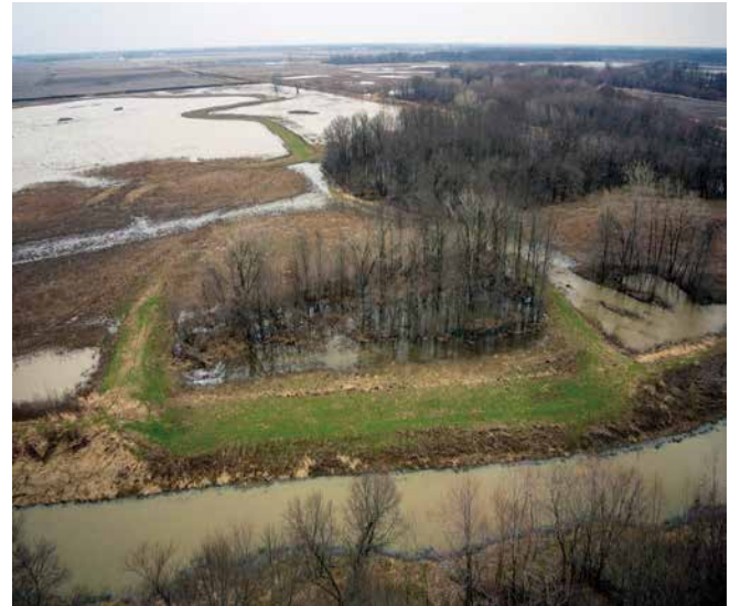
Figure 28b: Poorly designed floodway. Note the trapped water between the two training berms. These large pin oaks eventually died as a result.
