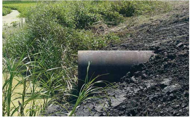
Figure 39: Smooth steel pipe installed in an existing berm.
