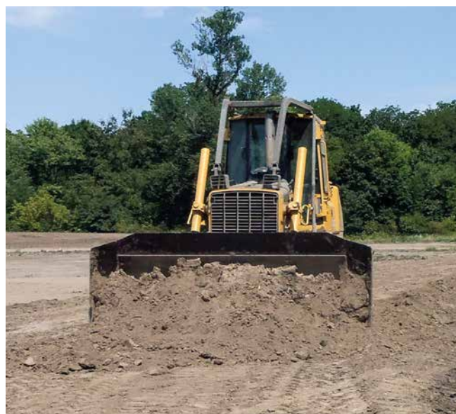
Figure 47: Bulldozer being used to “finish” a constructed berm.
