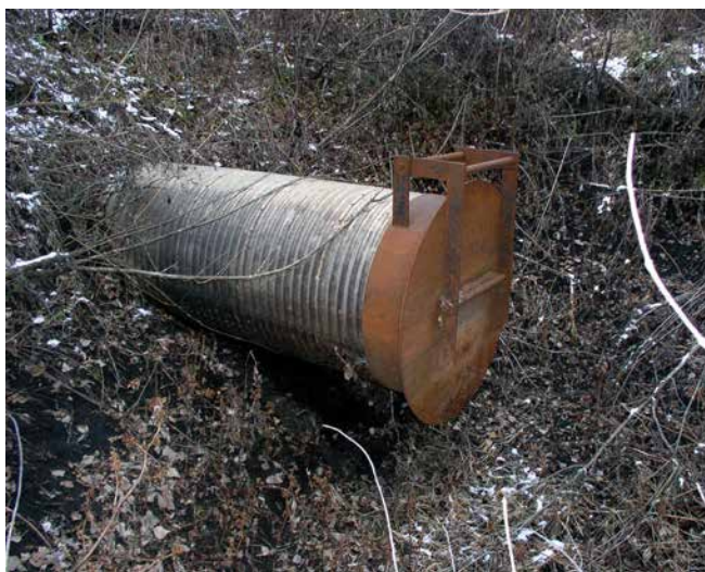
Figure 35: Flap gates, like the one pictured here, are often used to allow flood waters to enter a wetland pool prior to the overtopping of berms.
