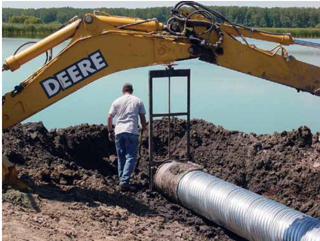
Figure 40: Corrugated metal pipe (CMP) being fitted with a screw gate.
