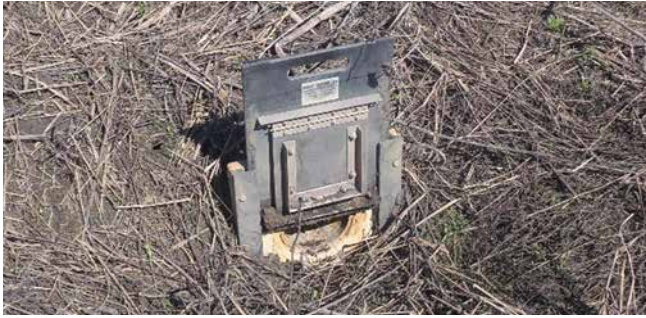
Figure 36: Slide gate with a built-in flap gate.
