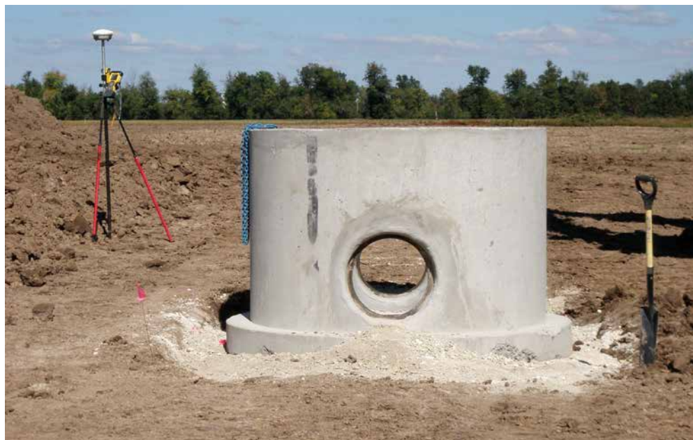
Figure 34: Round concrete manhole WCS prior to installation.
